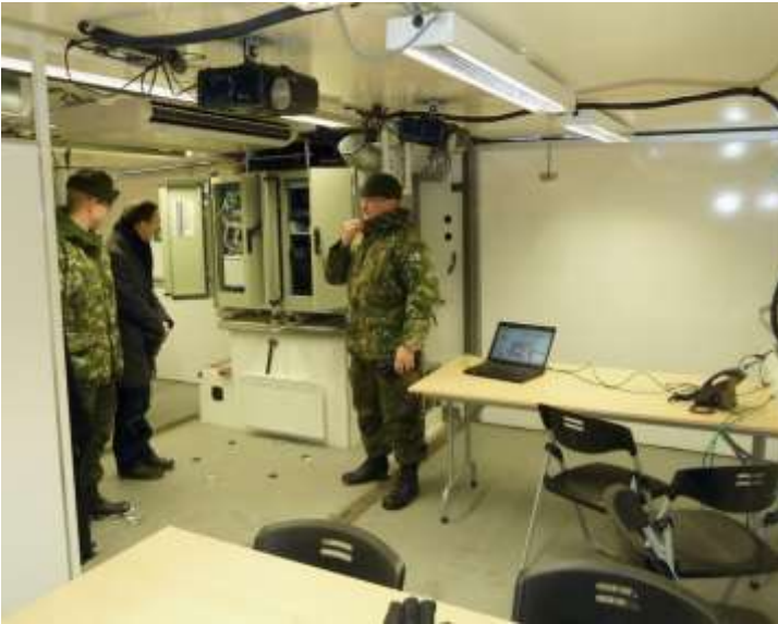
1521989 - Interior view of the expandable Command Post (CP) Module B under testing for the M18 system. CP Module B features workspace for up to 16 operators and has a set-up time of 30 minutes once deployed. Visible here are the communications cabinets with switching/routing and power electronics, as well as multimedia projectors and VoIP terminals. (IHS/Peter Felstead)
